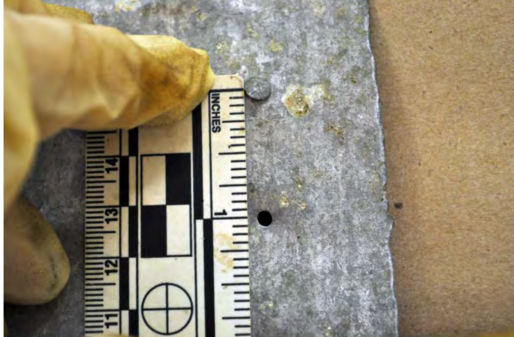
Figure 4: Smaller rivet holes were 1-inch apart. The intact rivet is shown.
